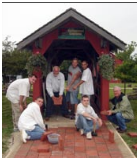
The crew lays down more bricks.
